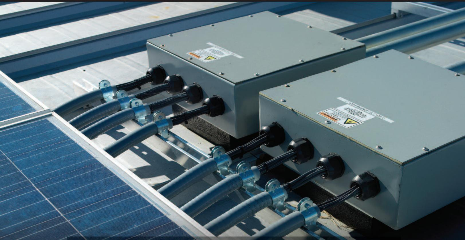
Solar Panel Array and Solar Masthead® II Cordgrips and Heyco-Flex™ I Conduit
